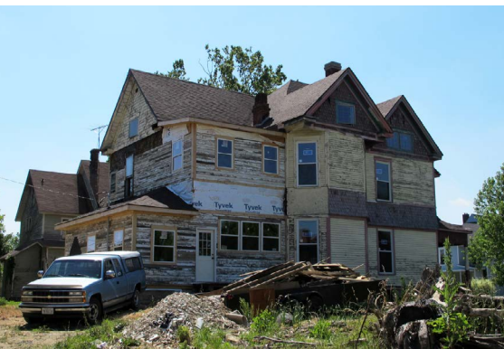
Rehabilitation activity in Muncie’s Emily Kimbrough National Register Historic District.
